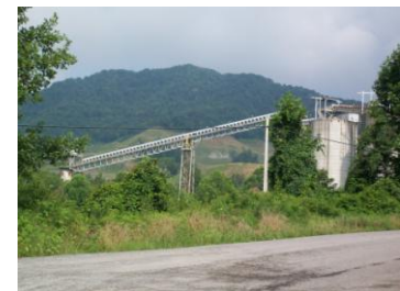
Keokee Mine Site
