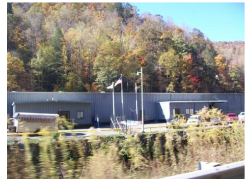
CONSOL Mine Rescue & Training Facility
