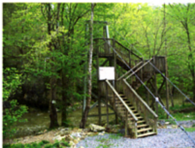
Suspension Bridge across Clinch River
