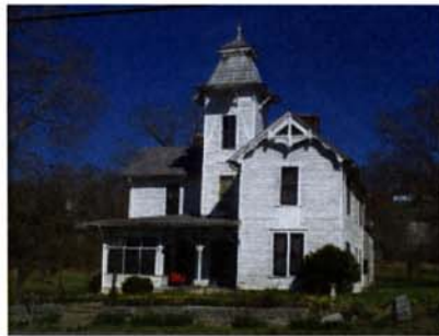
Historic home on VA 58 in Jonesville.
