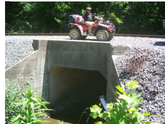
2) Tunnel along route goes under the railroad tracks is a unique feature along the route.
