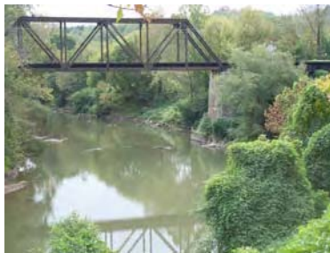
Warfield Railroad Bridge
