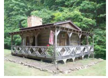
Existing one-room cabin
