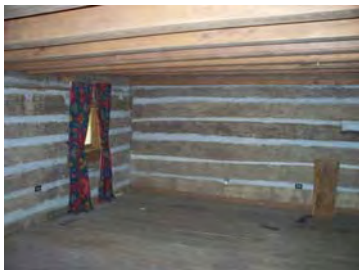
Interior view of a room
