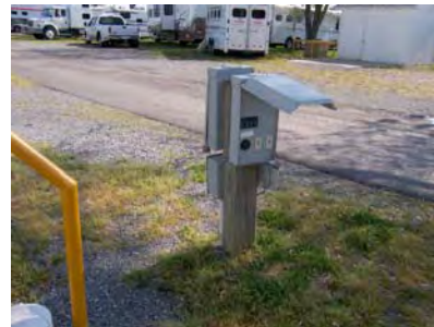
Double electric pole
